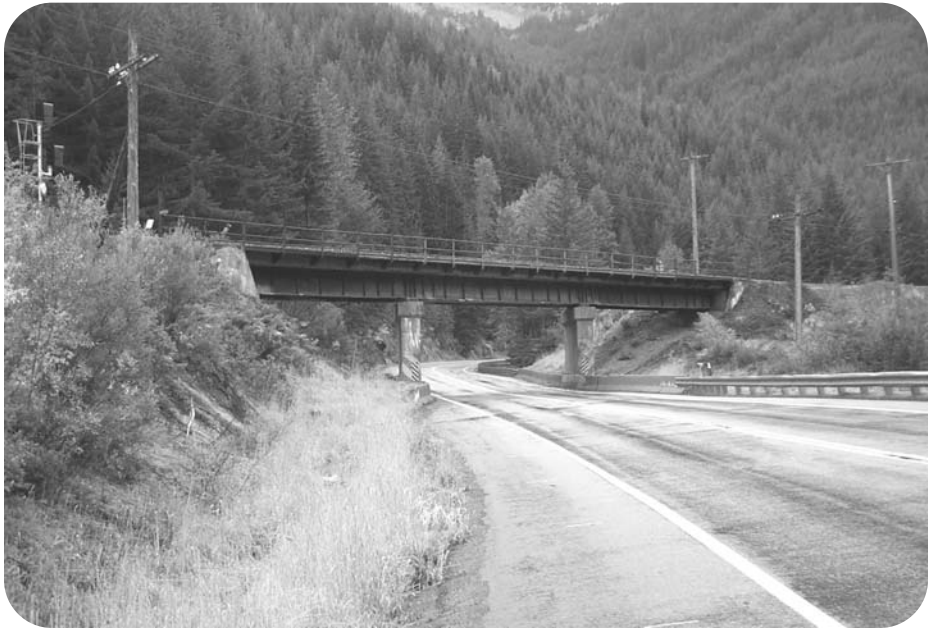
[Top] Sleeping with company! [Below] 5 feet under railroad tracks
